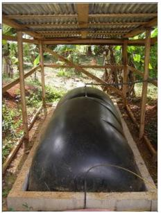
above. the biogas is then trapped by a large plastic balloon that hovers over the tank. Then, in the middle of the plastic, PCV tubing connects the biogas source to the kitchen, where the gas range (see picture at top of page) is ready to supply the alternative energy for cooking.
