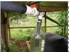
Then, you can prepare the PVC tubing frame that fits the plastic within the biodigester tank. To do this you can cut your 1/2" PVC tubing into pieces barely shorter than the measure of the inside of the rows of the cement block. The rest of the length (only a centimeter or two for each side) will be made up by the elbow connectors that connect the four pieces of tubing. Once the tubing is cut you can gently guide the tubing through the pockets made around the
