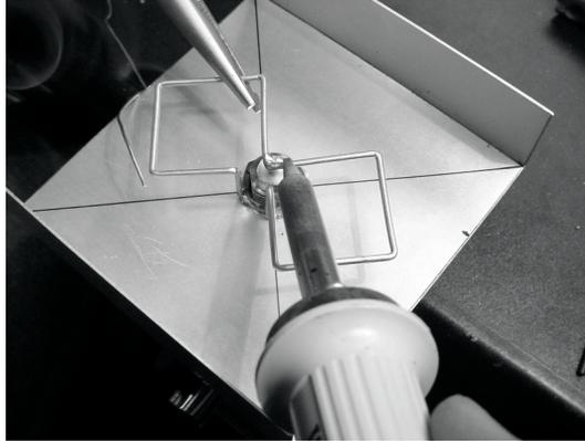
The procedure to fit the Biquad on the mounting bar may vary according to the shape of the original LNB fitting provided with the Parabolic Dish. It is usually round shaped, so it may be possible to use a rubber or plastic ring around the N connector to fix the Biquad in place.
