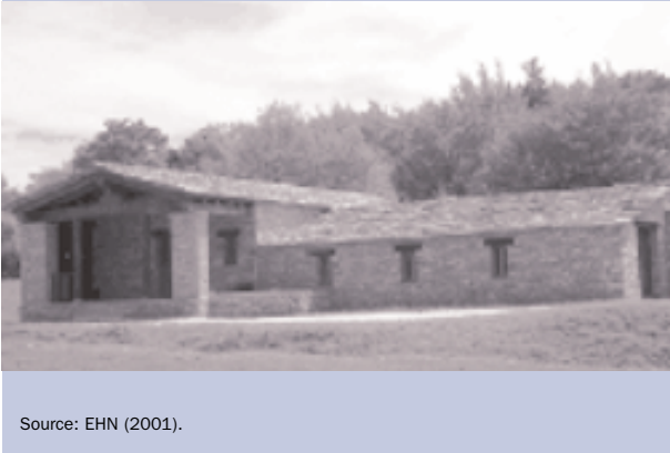
Figure 6.6: Substation, Ibargoiti Wind Park in Navarra (22 MW)
