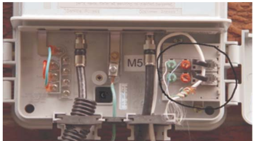
Splitter installed in a NID
