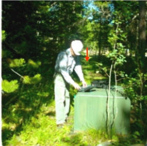
Setting-Up the Ground Tester Red arrow shows location of C2 probe.
