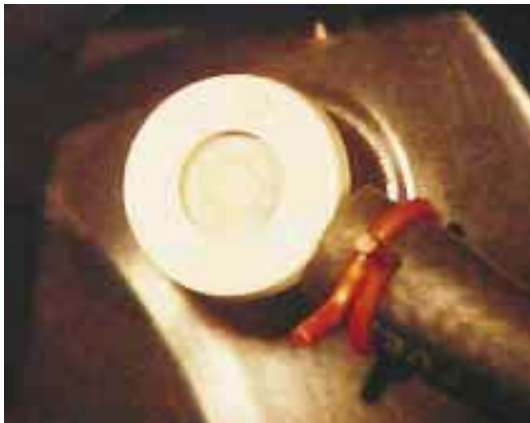
(Non-return valve on booster)
