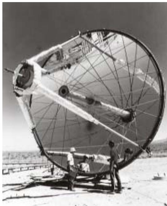
**Figure 16. 5200-sun, point-focus concentrator for a solar furnace. (Sandia National Laboratories/PIX01728)**
