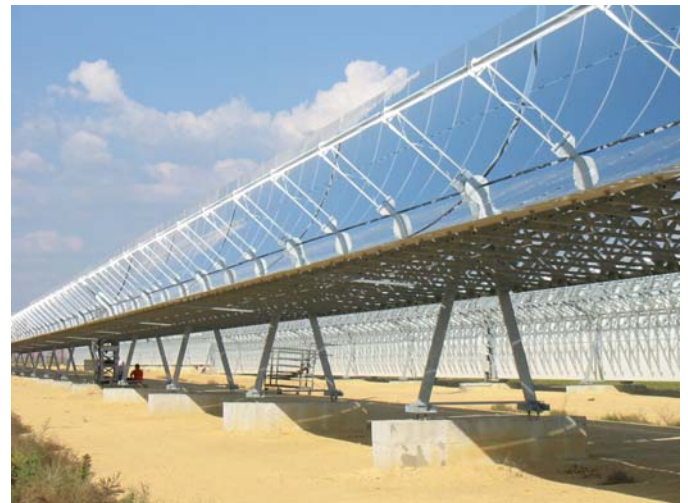
Figure 1: Solar Thermal Technology
