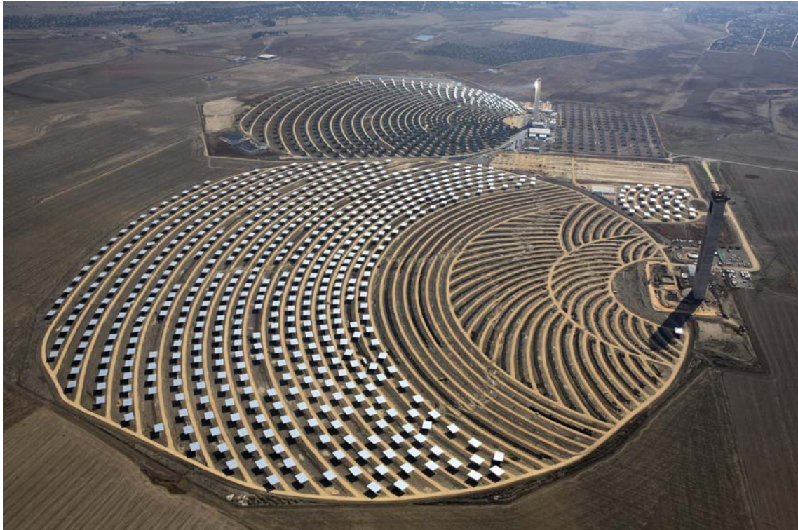
Figure 18. PS20 Plant under construction beside PS10
