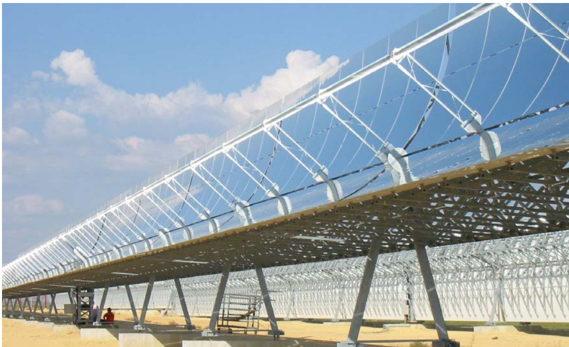
Figure 11: Abengoa Solar Trough
