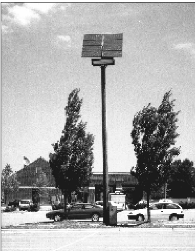
Figure 3: PV lighting at a park and ride facility in Raleigh, NC.
