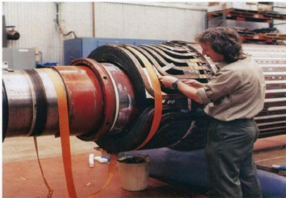
Repairs to the overhand insulation of this 200MW generator rotor were carried out by experienced tradesmen working on shift to ensure the earliest possible return to service.
