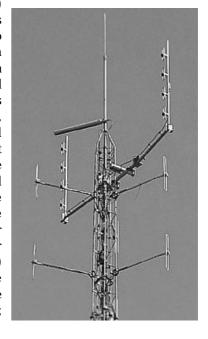
The folded dipole, being a variation of the simplest cage dipole, is one of the simplest 'skeletal' implementations of a "fat" antenna. Its terminal resistance can easily be deduced to a first order: see the box on the next page terminal resistance of a  $\lambda/2$  folded dipole =  $4 \times 73 \Omega$  for my own effort. I must admit I find the, different, explanations of this provided by Kraus [47], Page [48] and others difficult
