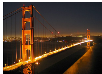
s / The Golden Gate Bridge's roadway is held up by the tension in the vertical cables.
