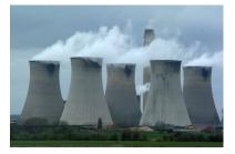
Large cooling towers, like the ones seen in power stations, are called **Natural Draft** towers. Standing at about 130m high, they are huge "chimneys" which create an updraft of air which cools the water as it falls down the inside of the tower. Natural draft towers do not contain any fans to drive the air flow.
