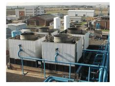
**Forced draft** cooling towers contain large fans which force air through a smaller tower. The photograph shows four box-like towers that are used to cool water in many industrial sites. These are also the types of cooling towers that may be seen on office blocks where they are part of the air conditioning system.
