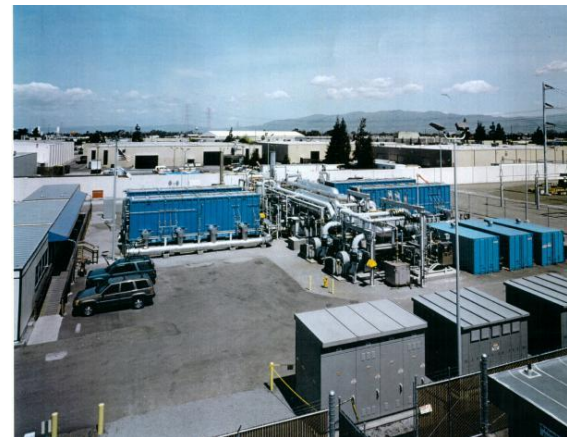
Energy Research Corporation's 2MW MCFC power plant demonstration in Santa Clara, California
