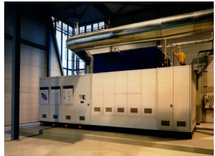
SOFC power plant built by Siemens Westinghouse
