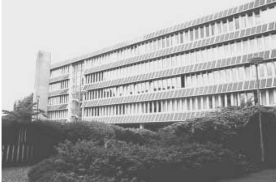
Figure 15.11 Example of facade integration of photovoltaics. The photograph shows the 40 kWp PV façade on Northumberland Building at the University of Northumbria. The PV array is integrated into the rainscreen overcladding. This system was installed in 1994 and is one of the early examples of façade integration (photograph courtesy of University of Northumbria).
