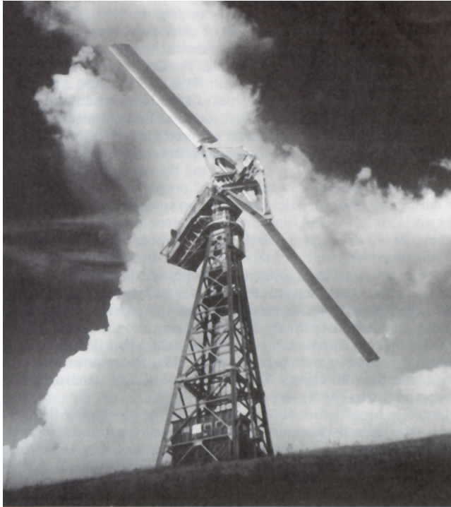
Figure 2.1: The 1.250 MW Smith-Putnam wind turbine. Reproduced from [37].
