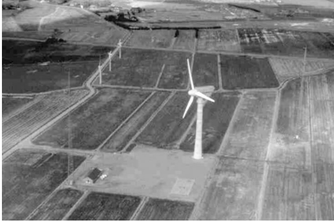
Figure 5.7: The Tjæreborg wind turbine. Reprinted from [20].
