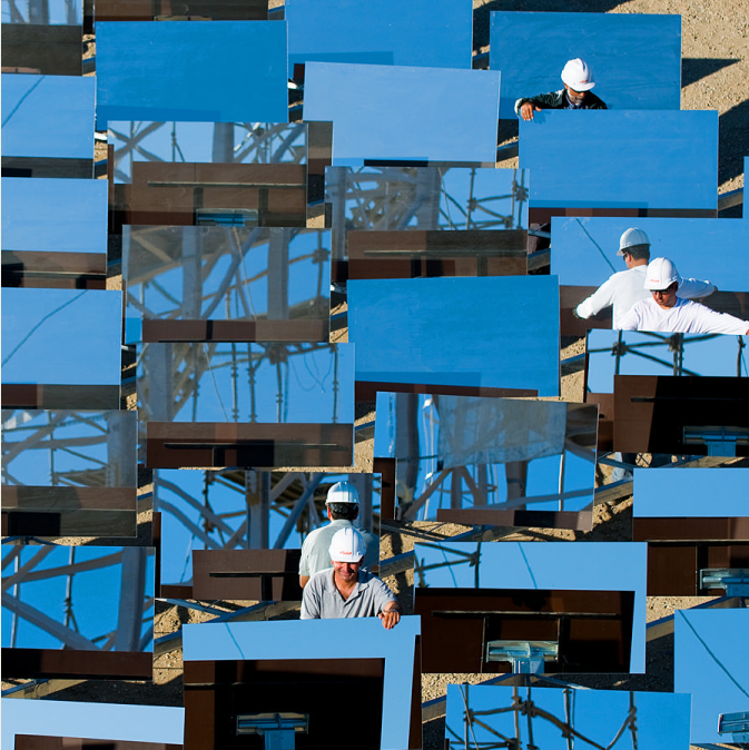
eSolar technicians configuring a point focus mirror array.
