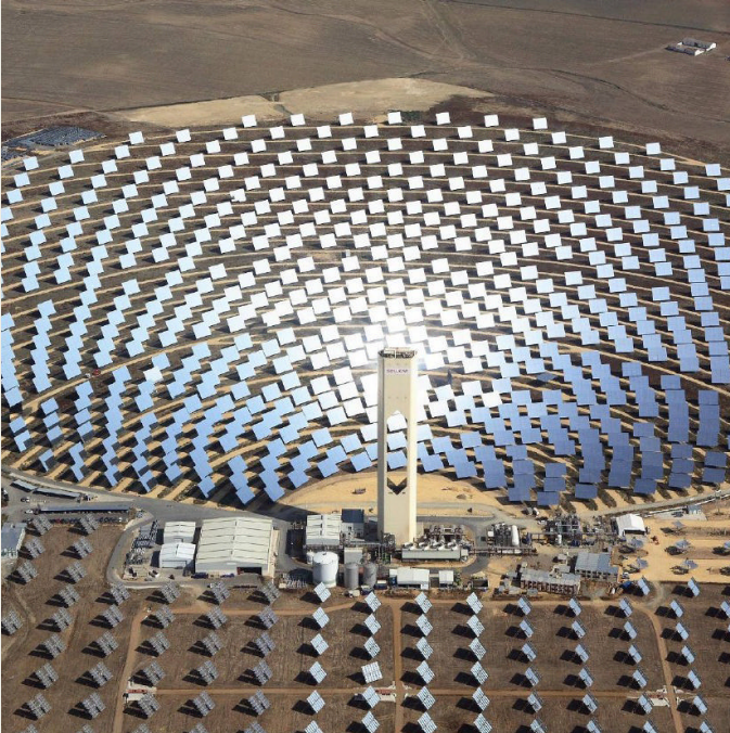
Europe's first commercial concentrating PS10 solar power tower is operating near the sunny southern Spanish city of Seville. The 11 megawatt solar power tower produces electricity with 624 large movable mirrors called heliostats.
