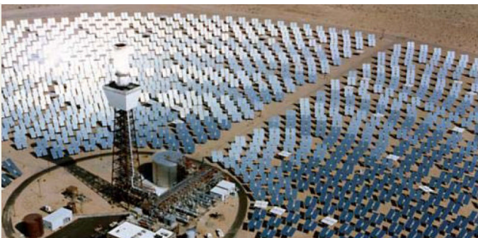
Point focus: The Solar Two project in California USA uses a field of mirrors to focus solar energy onto a central boiler to produce steam and electricity. (Photo courtesy NREL)
